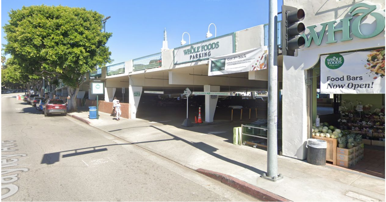
3. View looking northeast at subject site's parking garage.
